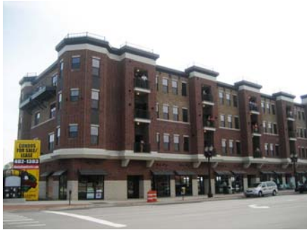
The Stadium District.
